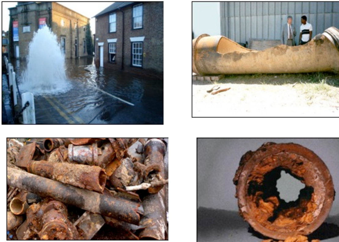
Figure 31: Broken water mains.
