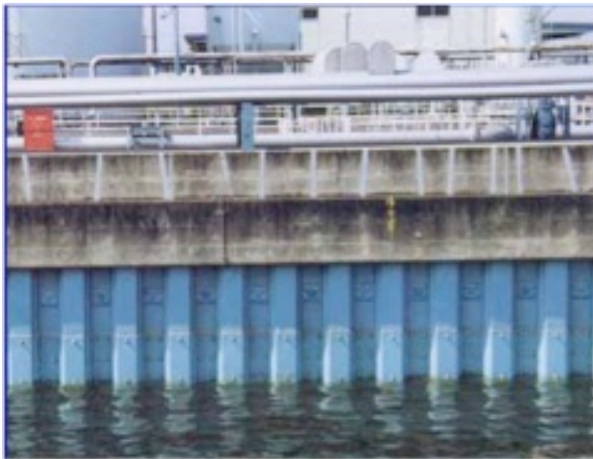
Figure 23: Underwater and splash zone coating. 29
