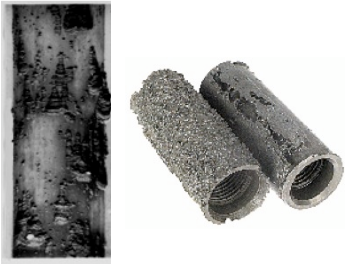
Figure 13: CO 2 corrosion of piping.
