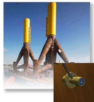
Impressed Current Cathodic Protection (ICCP) for Offshore Wind
